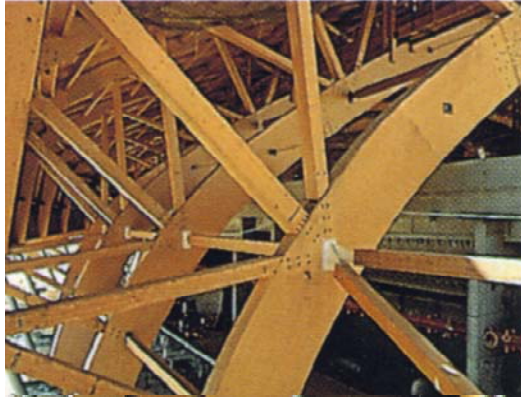
Figure 3: Arc treillis (Lisbonne, 1998)
