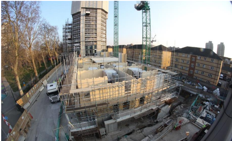
Figure 6: Installation Newington Butts
