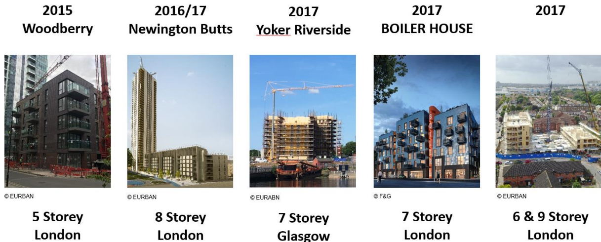
Figure 3: EURBAN Multi Storey Projects 2015 – 2015 © EURBAN Limited
