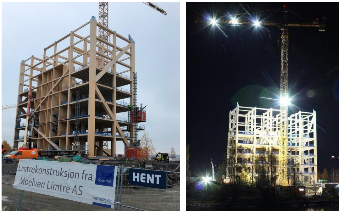
Figure 13: Images from the building site October 26, 2017
