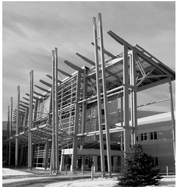
Figure 8: Exterior entrance glulam framing
