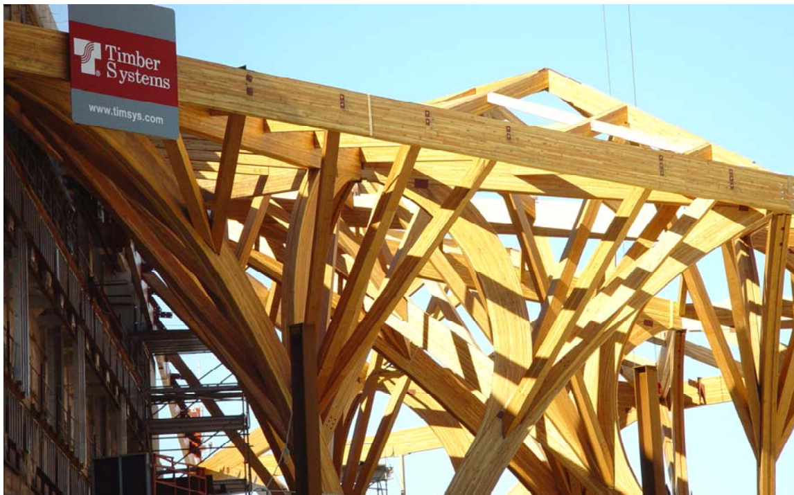
Figure 10: View of partially installed glulam atrium framing
