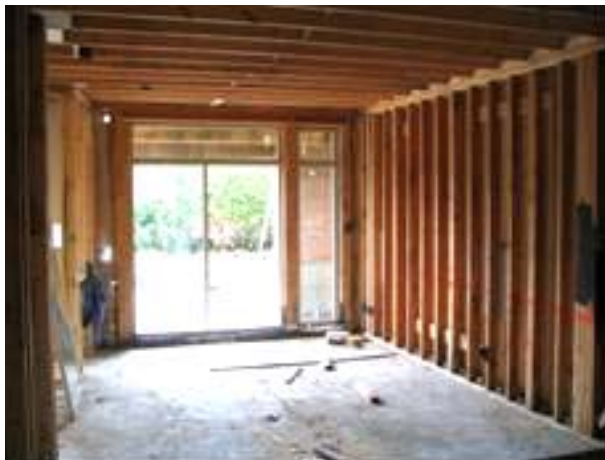
Figure 7, 8, 9 and 10: North America wood-frame construction
