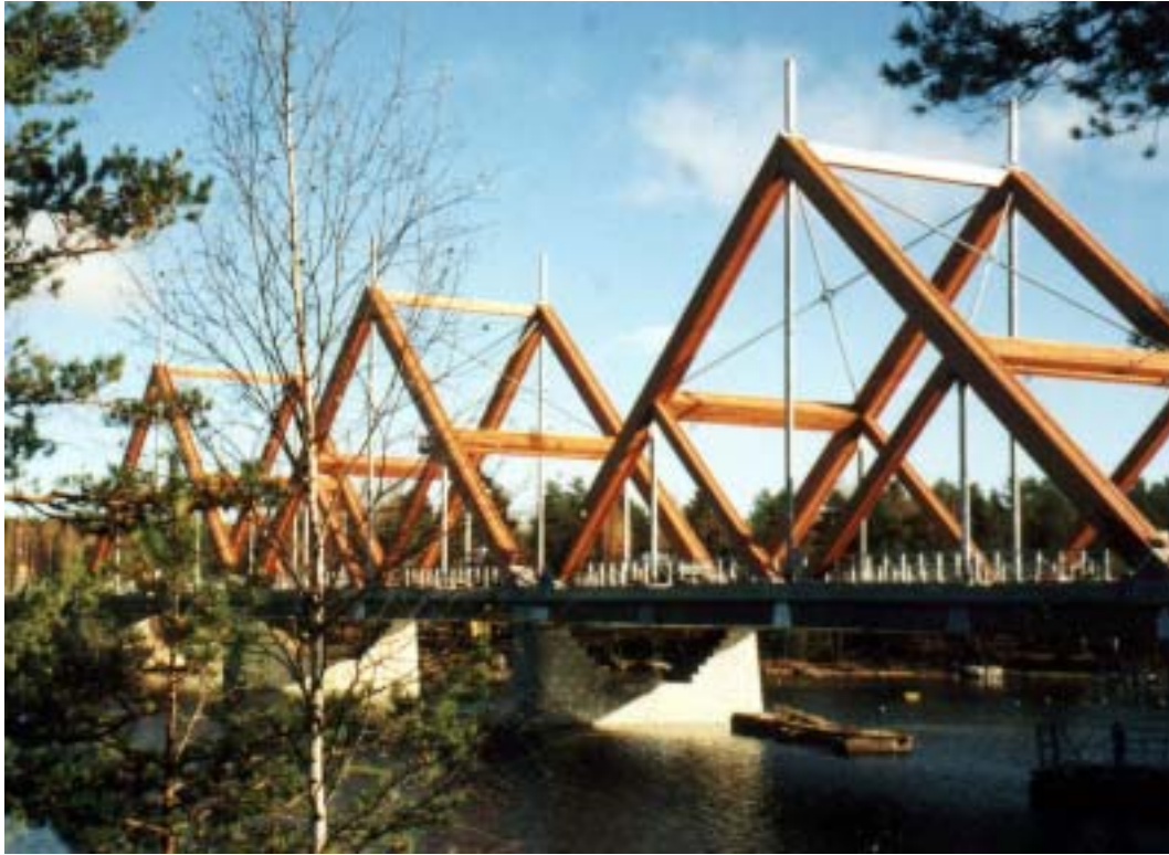
The Vammala Bridge
