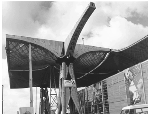
Figure 14. The leg and large girders are assembled from two box-beams. The length of the girder is 18.6 m.
