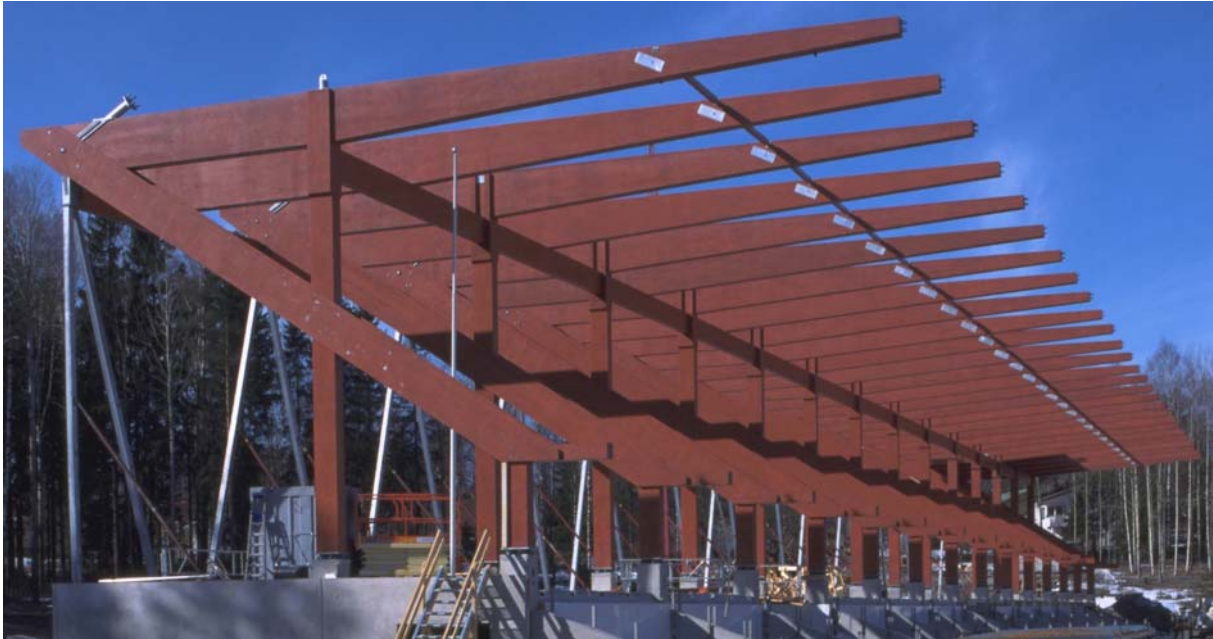
Figure 16. The wooden frame of Silva Stadium in Vantaa, Finland.
