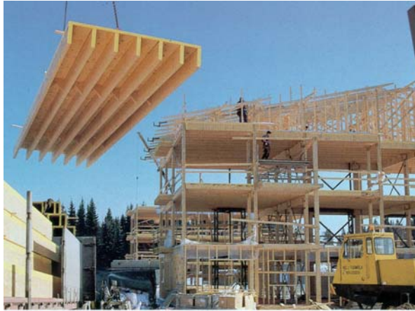
Figure 4. Stress skin elements were erected rapidly on the building site
