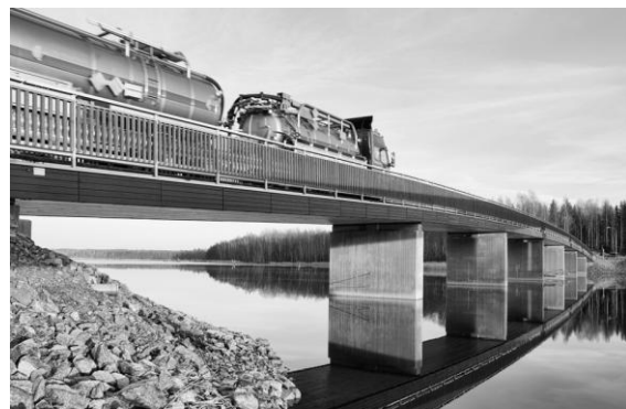
Figure 8: Road Bridge Iggesund in use
