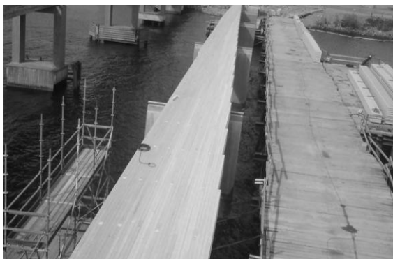
Figure 7: Road Bridge Iggesund during assembly
