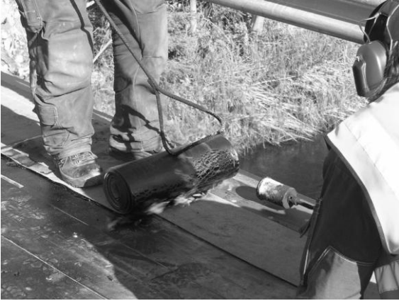
Figure 14: Watersealing at deck edge
