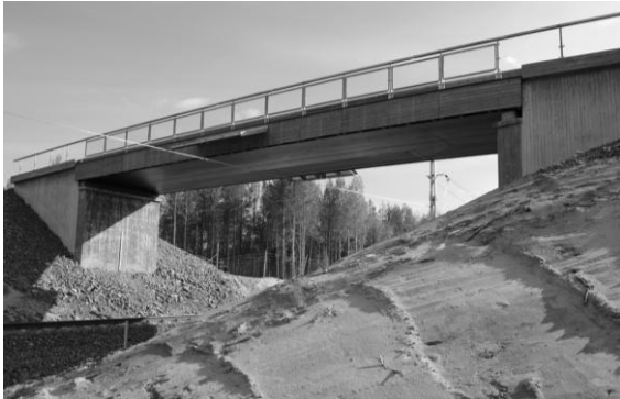
Figure 5: Road Bridge Hataträsk, veiwedfromrailroad
