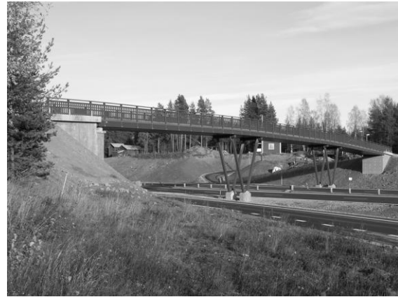
Figure 10: Pedestrian Bridge Iggesund in use
