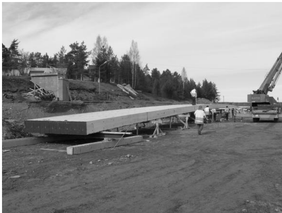
Figure 9: Pedestrian Bridge Ostvik, during assembly
