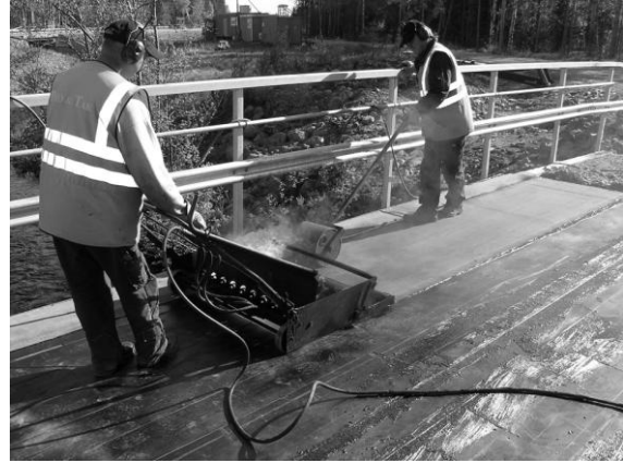
Figure 15: Watersealing on top surface of deck
