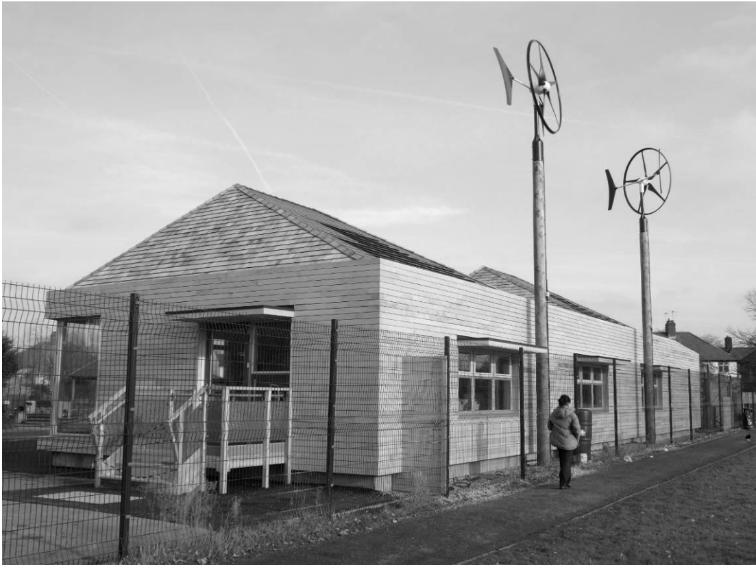
Abbildung 11: Roe Green Primary School © dm3 Architecture
