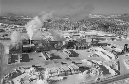
Figure 3: Usine de Chantier Chibougamau
