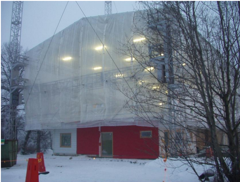
Picture 7: Weather protection with assembly platform at Älvsbacka strand in Skellefteå
