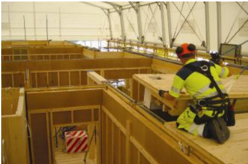
Picture 2: Assembly of floor structures at Limnologen in Våxjö
