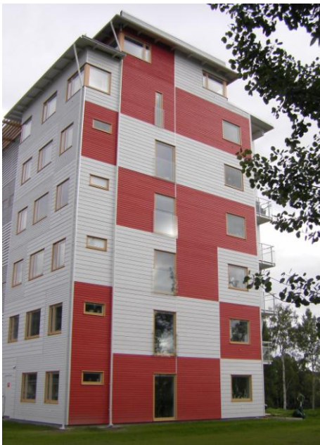
Picture 5: Älvsbacka strand in Skellefteå is a six-storey residential building
