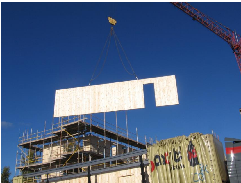
Picture 1: Wall unit on its way at Hyttkammaren in Falun
