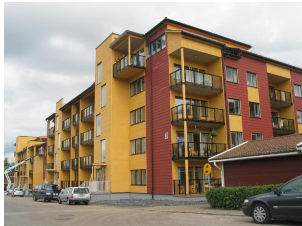
Picture 6: Hyttkammaren in Falun is a 4-storey residential building
