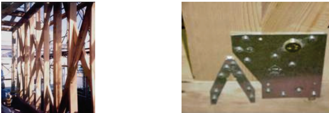
Figure 2: Japanese post and beam construction
