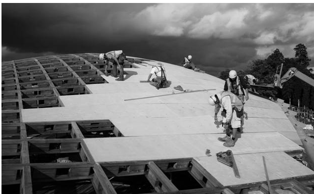
Figure 23: The Plywood covering
