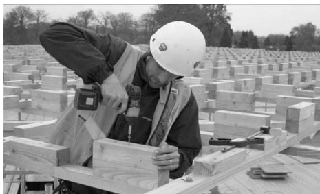
Figure 26: Fixing shear blocks Photo: Buro Happold / Adam Wilson
