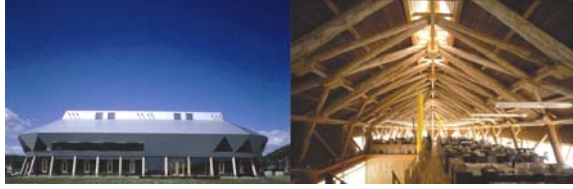
Figure 11: Oketo national district forest office, Hokkaido 1993
