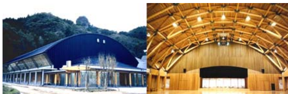
Figure 28: Yamakuni municipal Misato primary school gymnasium, Oita 2002
