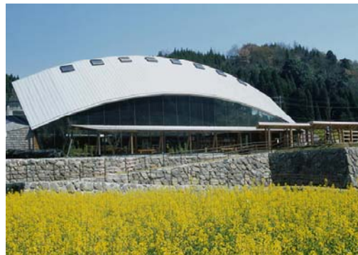
Figure 3: Roadside station, Asaji town, Oita 1999
