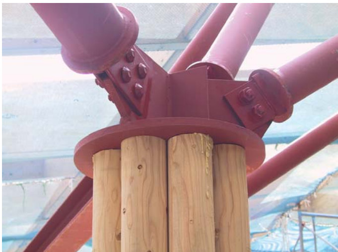
Illustration 7: Top joint of Bundled pillars
