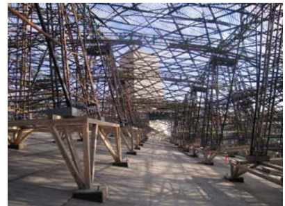
Illustration 11: Bamboo construction (inside Cage) on the roof
