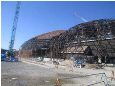
Illustration 9: Bamboo Cage, construction in progress
