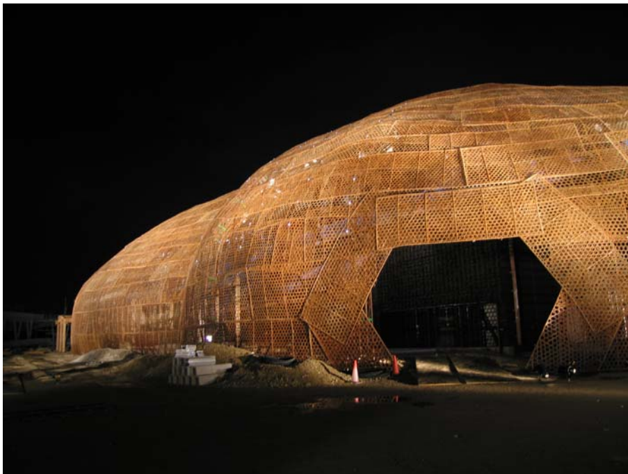
Illustration 20: Japan Pavilion Nagakute at night (Under construction)
