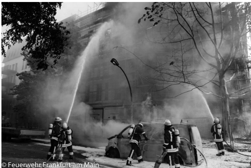
Abbildung 1: Polystyrol-WDVS-Brand in Frankfurt
