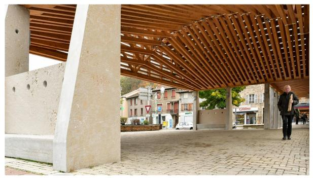
The Vinsobres childcare building, with massif wood structure, straw insulation and earth and lime plasters on the walls.
