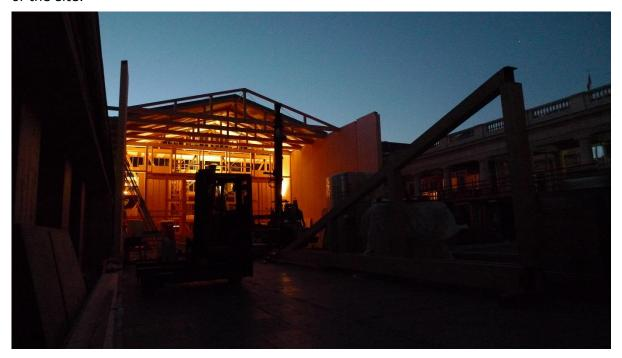
The fact of bringing prefabricated roof panels already waterproofed made it possible to advance each day by more than 120 m2 (hundred twenty squared meters) covered and closed.
