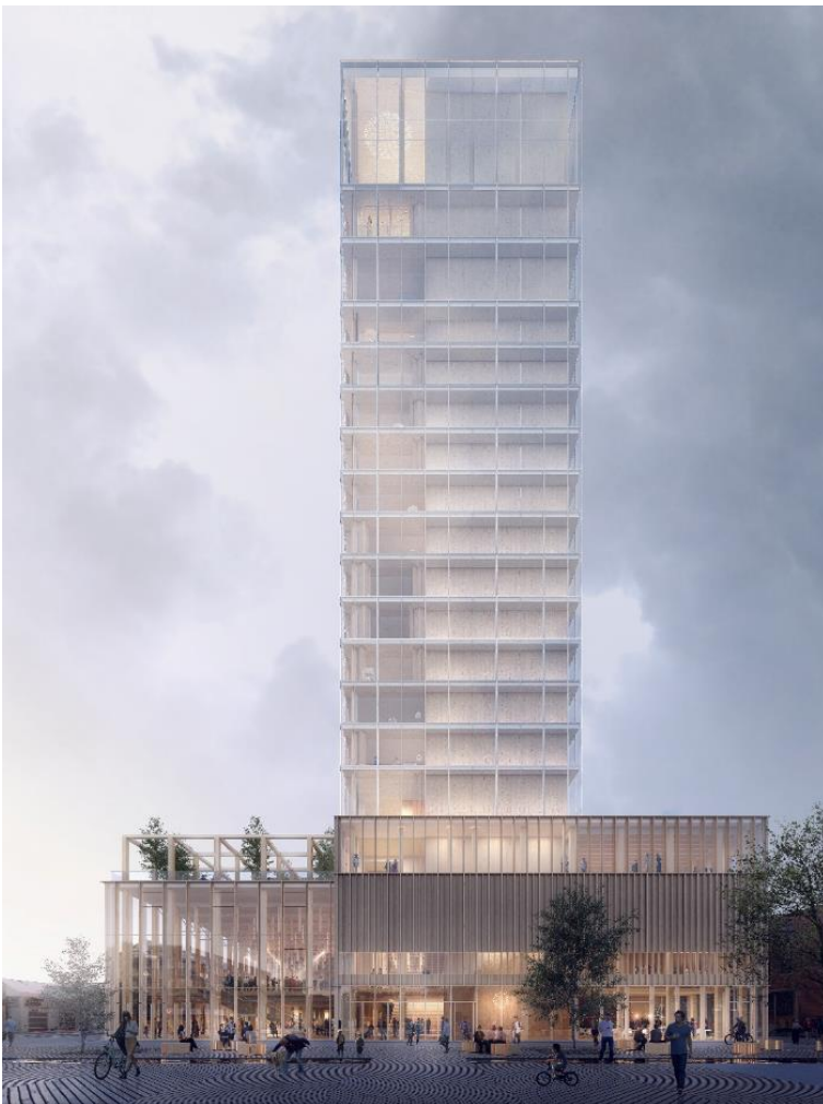
Figure 9: Stabilizing timber shafts visible through the hotel double-skin façade. (Image by Luxigon)
