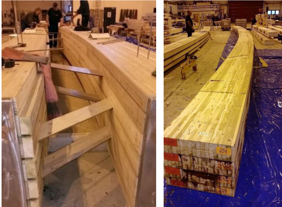
Figure 13: Pre-assembly of the arches in the glulam factory
