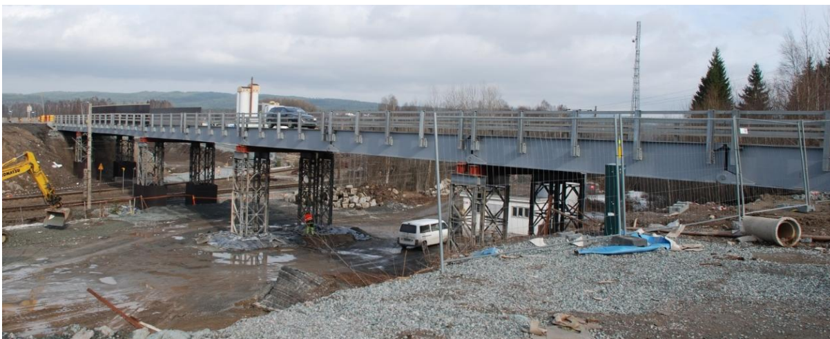
Figure 16: Interim bridge east of the existing bridge
