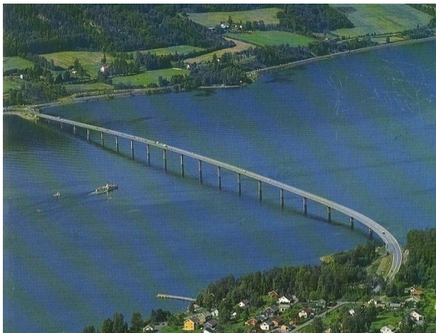
Figure 22: Overview of 1st Mjøsa Bridge
