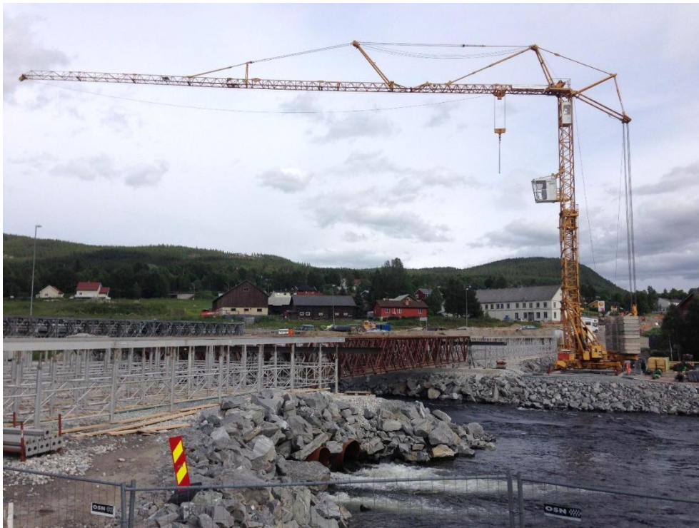
Figure 11: The construction site
