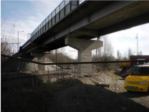
Figure 15: Existing concrete/steel bridge
