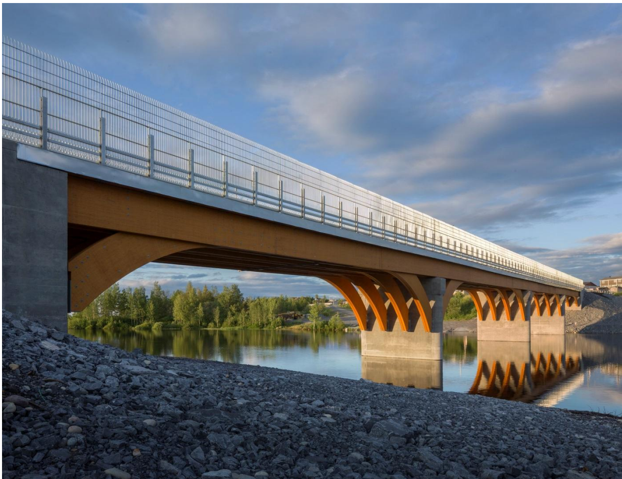
Figure 16: View of the bridge from east bank
