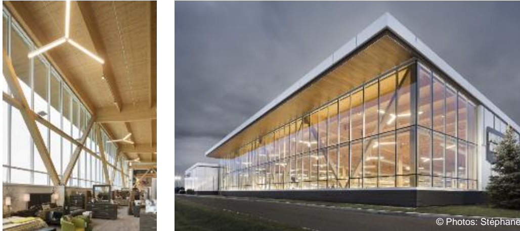
Figure 6: V-shaped columns on the building's facades
