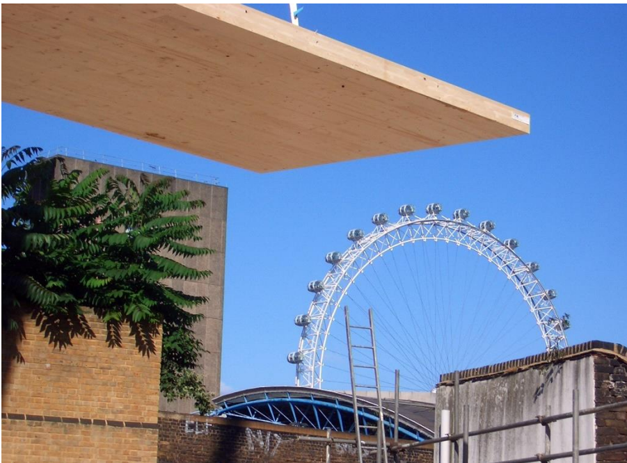
Figure 2: Carlisle Lane Lofts, Picture © EURBAN
