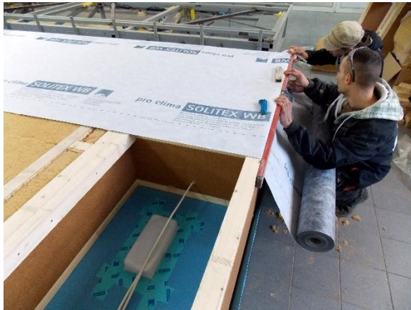
Figure 12: Sealing the walls and ceiling.
