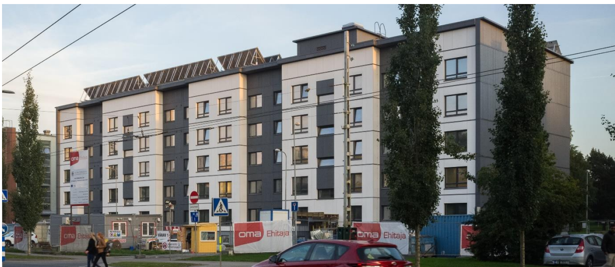
Figure 3: Well insulated building envelope with onsite energy production is needed for nZEB.
