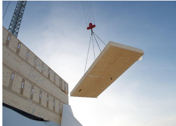
LVL R and LVL X: pre-fabricated floor elements. Photo: STEICO
