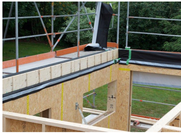
LVL X: rimboard in floor construction. Photo: STEICO
