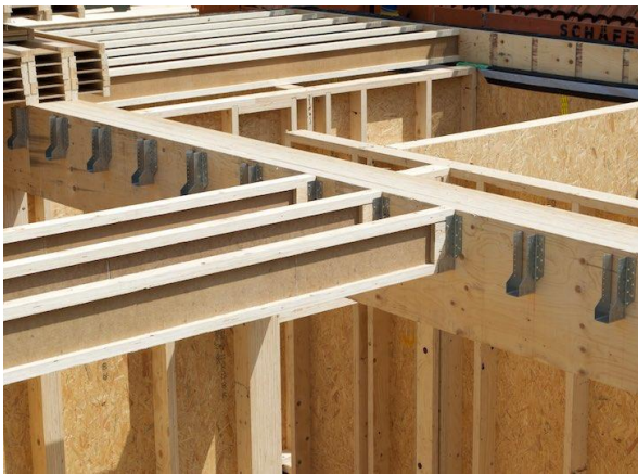
LVL R: primary beam in floor construction. Photo: STEICO
