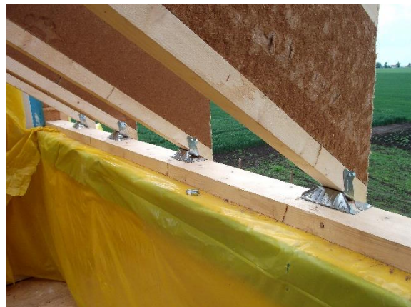
Pre-insulated I-joists: connection at eaves using variable pitch seat connector Simpson VPA. Photo: Szreder A.C.
