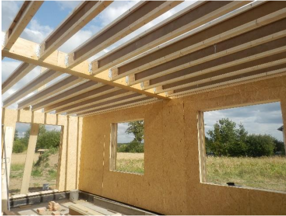
I-joists: secondary beams in floor construction. Photo: Hebelodom / STEICO
