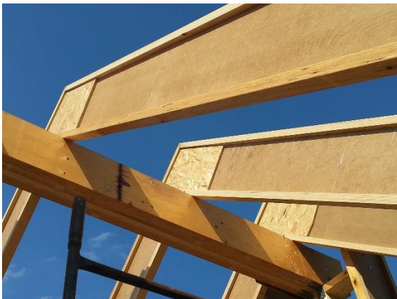
I-joists: rafters in roof construction. I-joists support on ridge beam made from LVL R Photo: Aleksandra Knychas / STEICO
