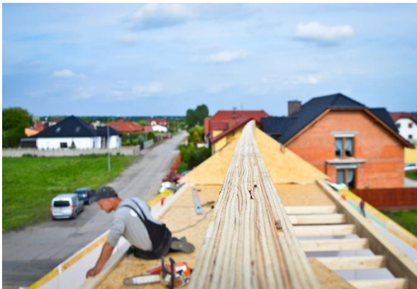
LVL R: ridge beam in roof construction. Photo: Genero
