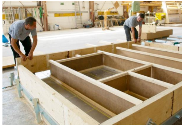
LVL R: top plates in walls construction. Photo: STEICO
