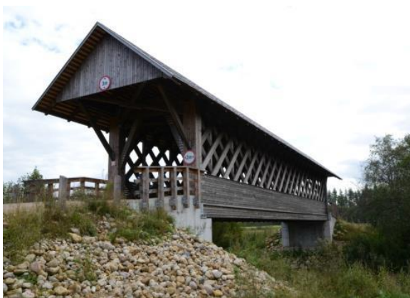
Figure 16: Järuska covered bridge.
