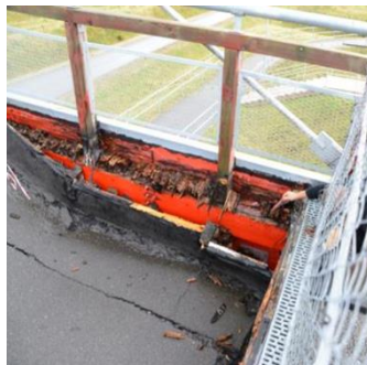
Figure 4: Collapse of the deck in 2014 due to completely rotten deck at supports.
