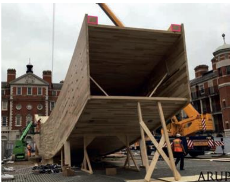
Figure 9: The Smile – Roof to wall connection
