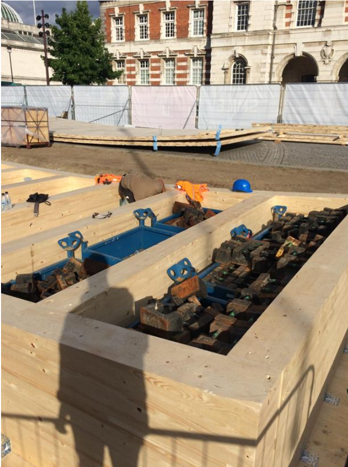
Figure 5: The Smile – Foundation counterweights
