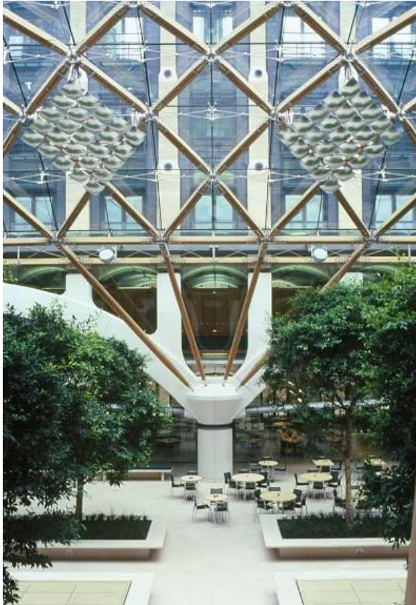
Figure 1: The courtyard roof of Portcullis House, London 2001
