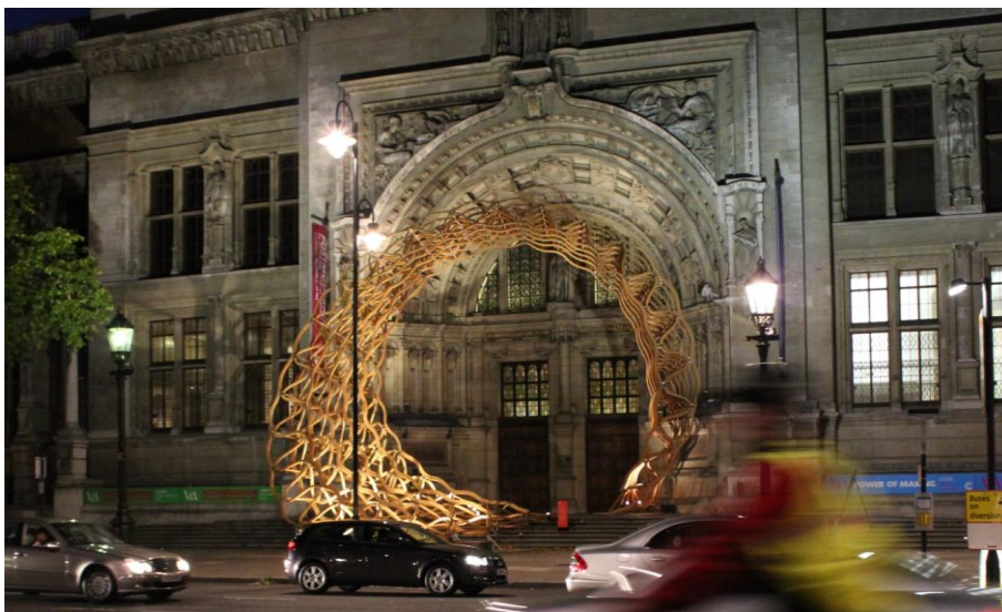
Figure 2: The Timber Wave, London 2011
