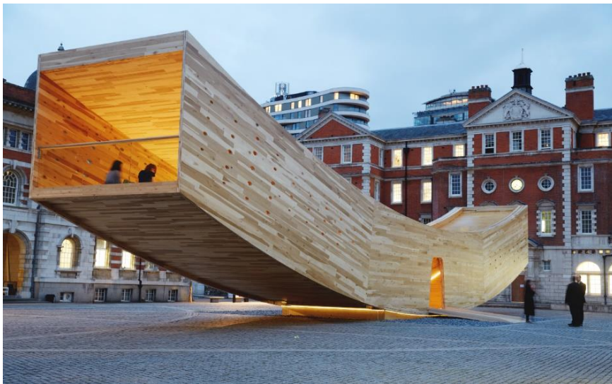
Figure 11: The Smile - Completed structure
