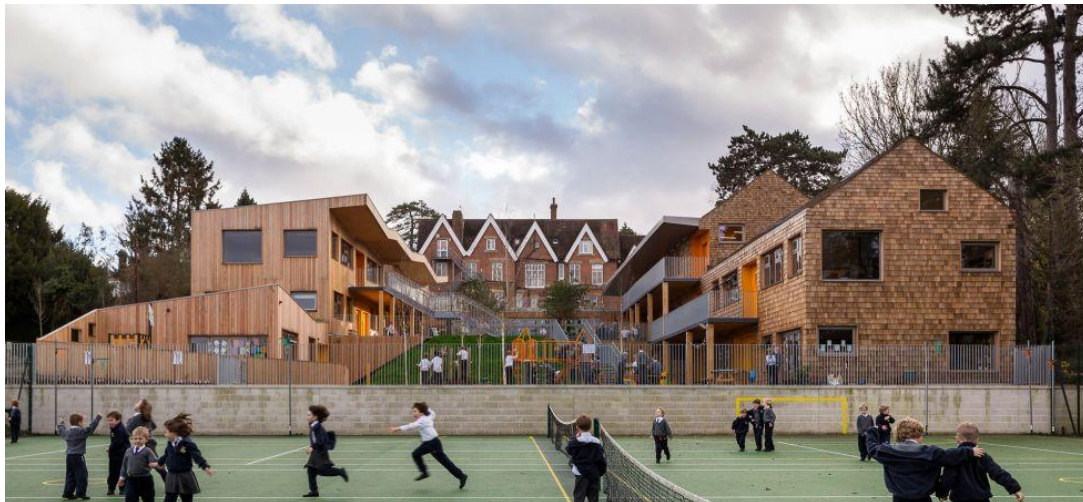
Image 4: Hawkins\Brown's recently completed Hilden Grange School was constructed from CLT. Image copyright Tim Crocker
