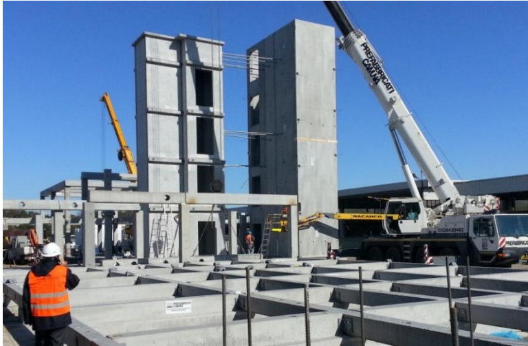
Figure 20: Concrete prefabricated structure
