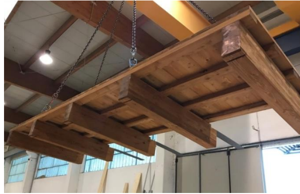
Figure 9: Construction of Xlam balconies in the factory.
