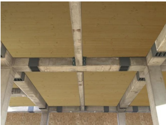
Figure 12: The correct material in the correct place: wood, concrete and steel.
