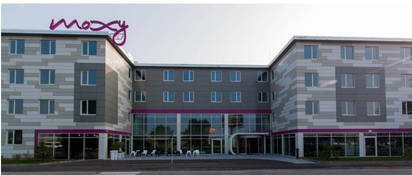
Figure 18: Moxy Hotel in Malpensa (VA)
