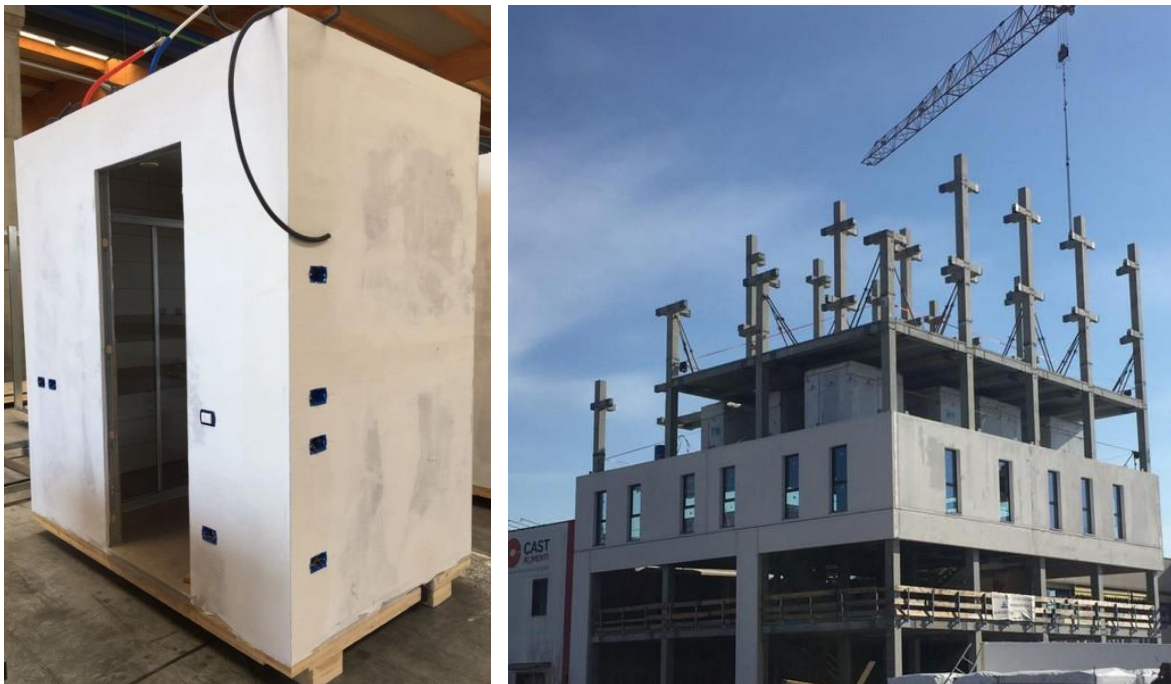
Figure 15+16: Prefabricated bathroom in the factory and site positioning.
