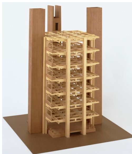
Tragwerkmodell Richards Medical Research Building (Quelle: MOMA)
