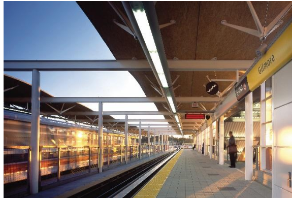
Figure 10: View from platform
