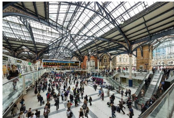
Figure 4: Liverpool St Station – London, UK – 1874
