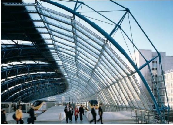
Figure 5: Waterloo Station – London, England
