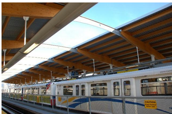
Figure 8: View from platform
