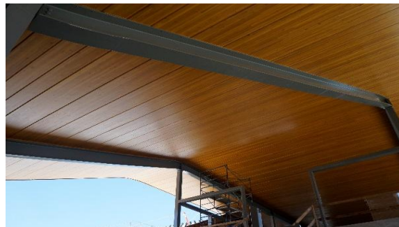
Figure 20: Interior view during construction
