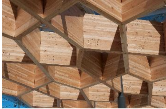
Figure 22: Close up view of roof structure
