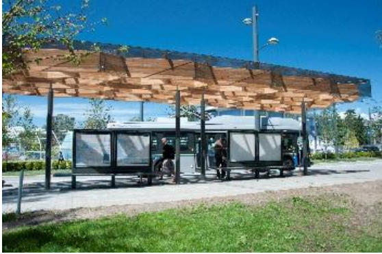
Figure 21: UBC transit shelter
