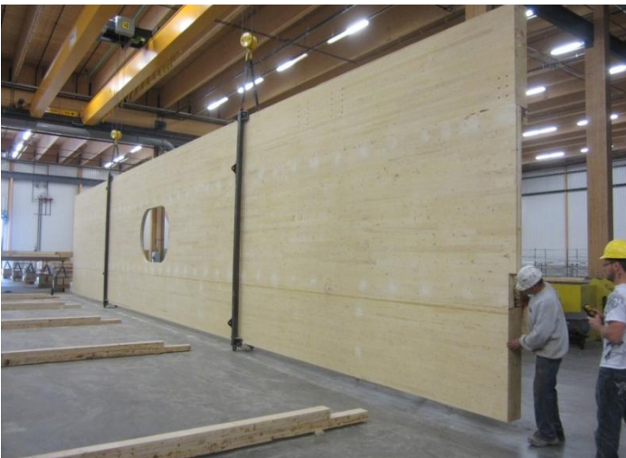
Figure 16: Fabrication of a principal beam, flipping of half section
