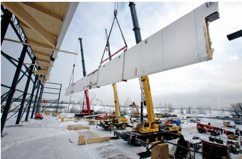
Figure 21: Installation of the second principle beam
