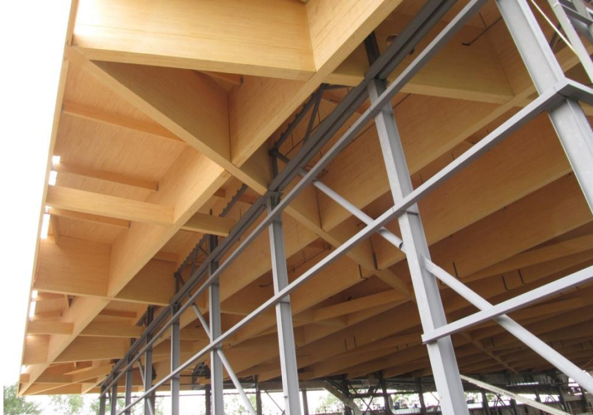
Figure 25: View of the completed of the cantilever roof structure
