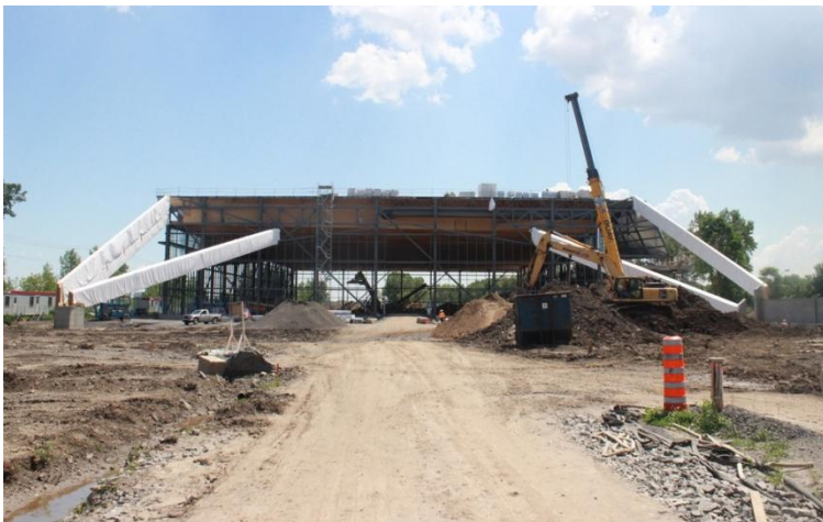
Figure 23: Installation of the "Shoulders"
