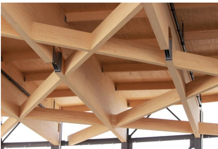
Figure 24: View of the completed roof structure
