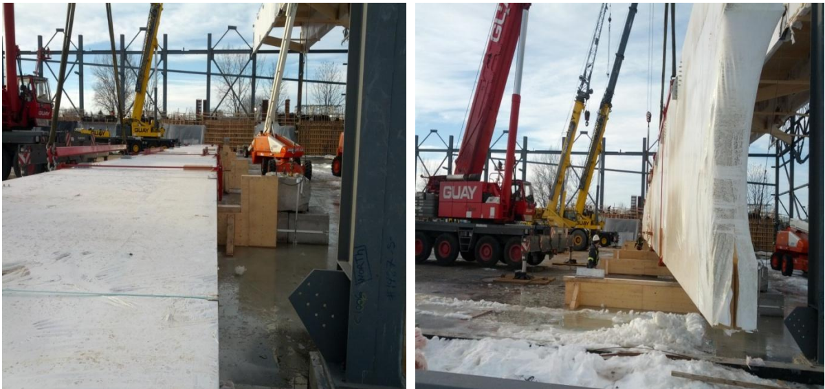
Figure 20: Temporary reinforcements (left) and flipping of the beam (right) [2]
