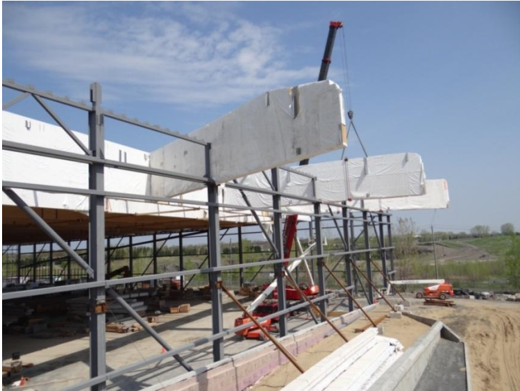
Figure 22: Installation of the cantilever beams
