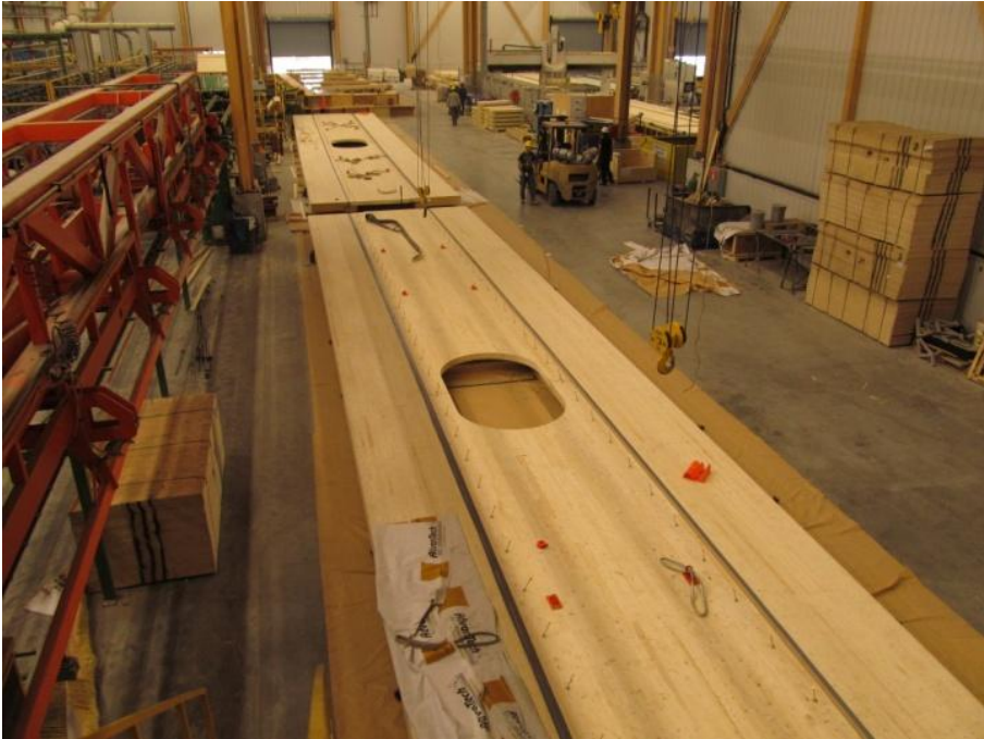
Figure 15: Fabrication of a principal beam
