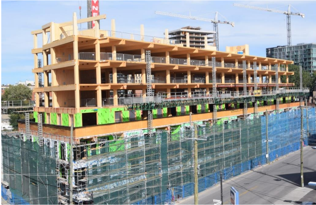
Figure 9: Installation of Arbora, Sept. 26, 2016
