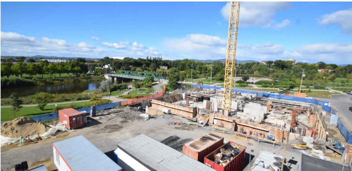
Figure 18: Foundation installation of Origine, Sept. 25, 2016
