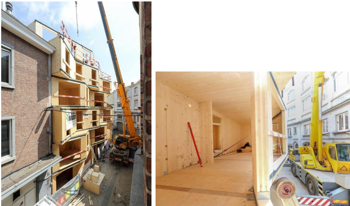
Figure 3 and 4: Ki-Etude housing construction site pictures by Pascal Themans
