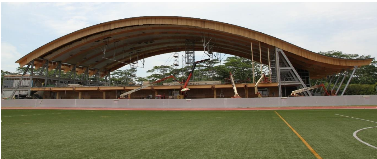
Figure 5: elevation view of the shallow shape of the arches of the Wave
