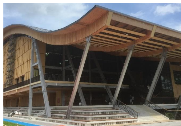
Image 7: steel A-frames providing support for the side hinge of the arches
