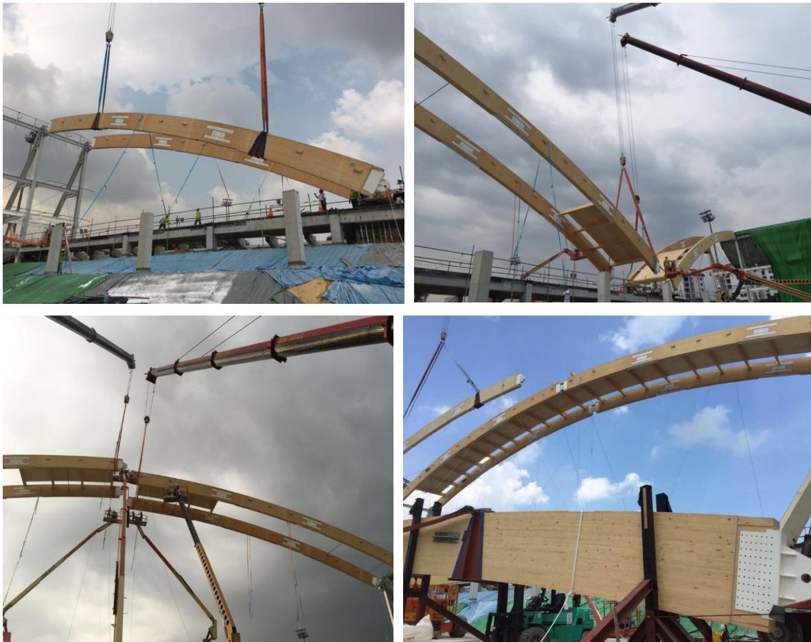
Image 16: launching of arches
