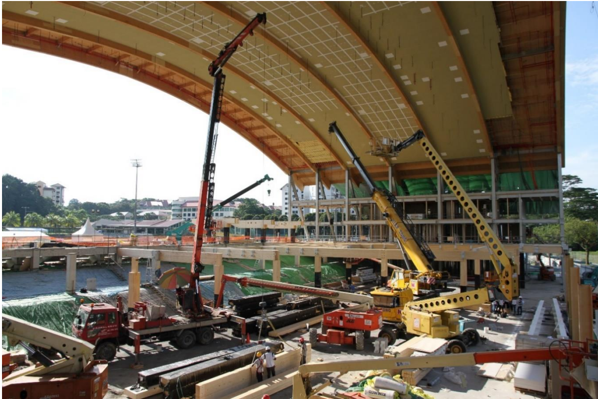
Image 18: phases of the erection sequence of the interior stories
