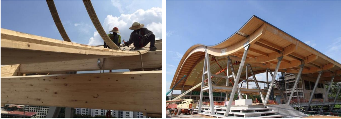
Image 14: CLT stiff diaphragm on the roof
