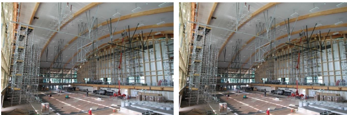
Image 19: main glulam coupled beams on the exterior façade
