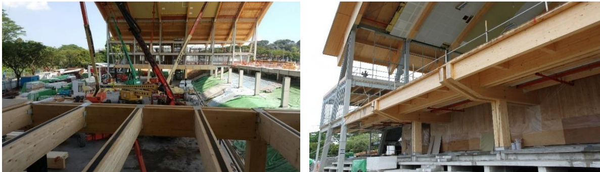
Image 19: main glulam coupled beams on the exterior façade
