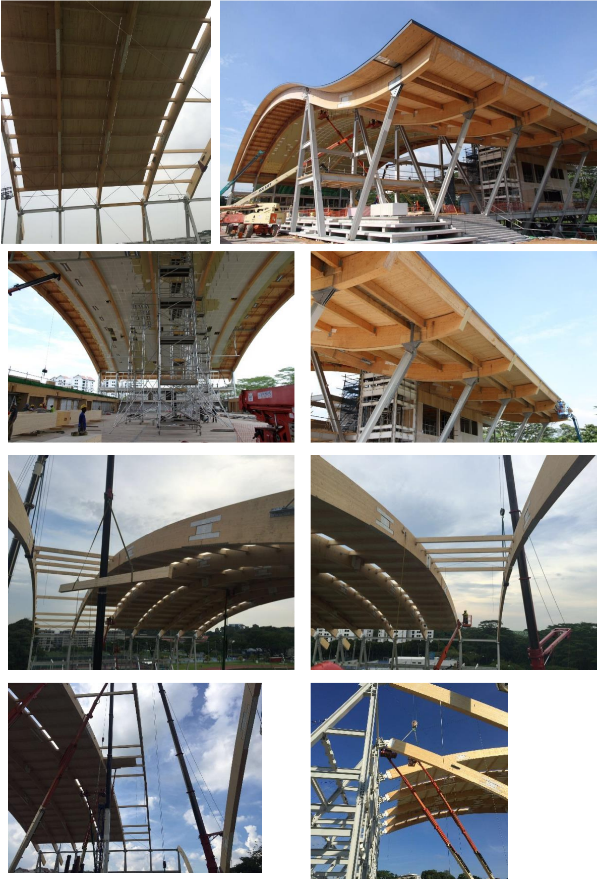
Image 17: following phases until completion of the arch system
