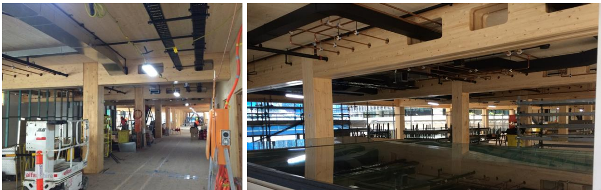
Figure 9: Beams in situ on site during installation of the services
