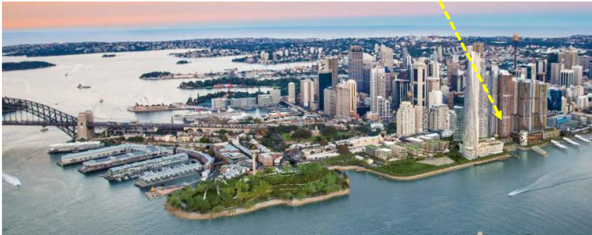
Figure 15: Location of International House, Sydney – Darling Harbour view
