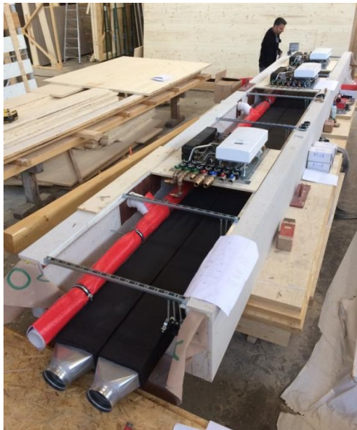
Images 9 and 10: Prefabrication and erection of the shaft with M&E installations
