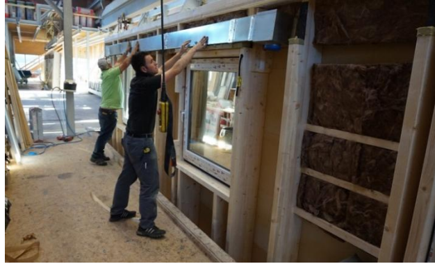
Images 5 and 6: Installation of ventilation ducts in the factory. Source: Gump & Maier GmbH
