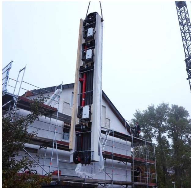
Images 9 and 10: Prefabrication and erection of the shaft with M&E installations
