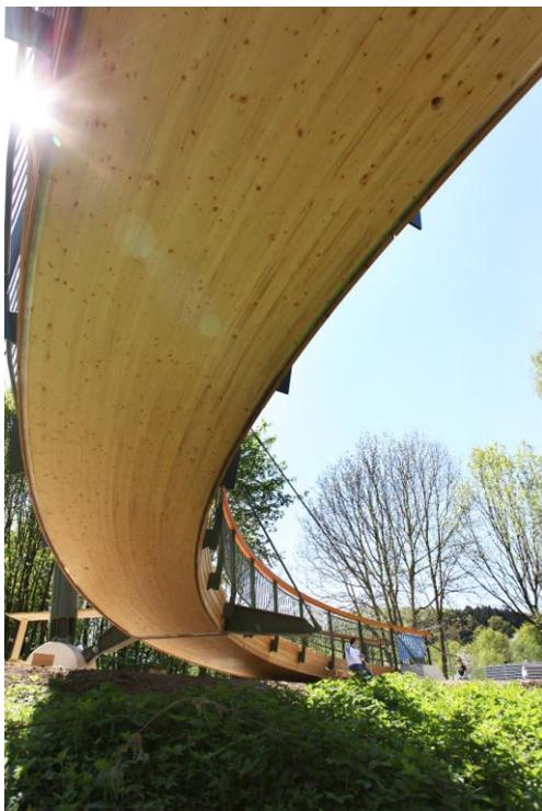
Figure 3: block lamination of twisted beams
