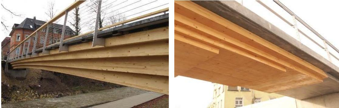
Figure 8: stepped block-laminated timber
