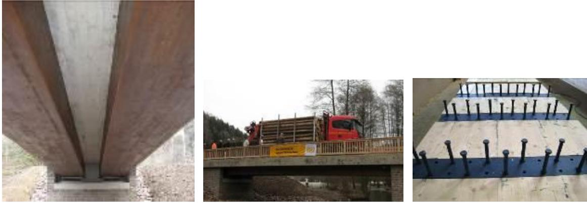
Figure 10: shear connection by head bolts
