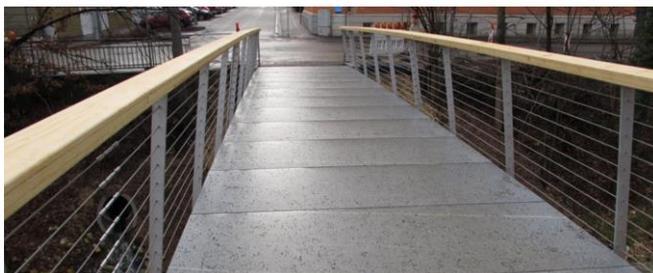
So, the combination of a carrying timber structure with granite as a bridge flooring material brings interesting prospects:
