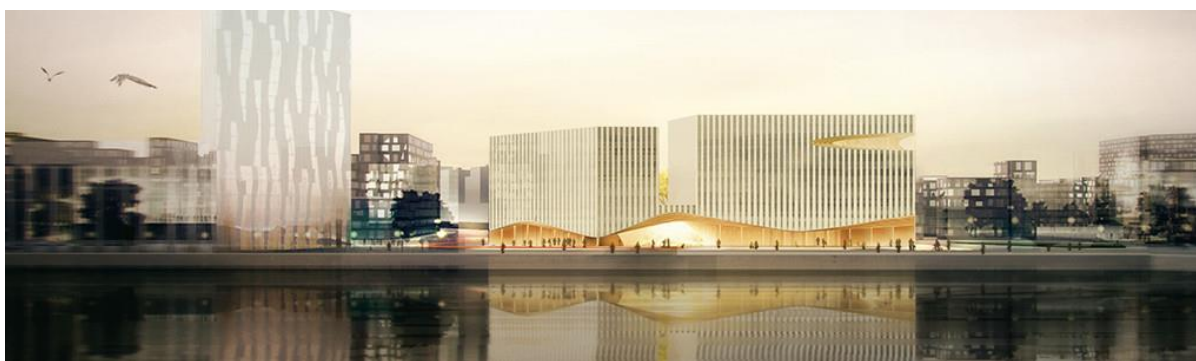
Figure 3: Wood City will be Finland's largest wooden quarter. Picture: Wood City/SRV Group
